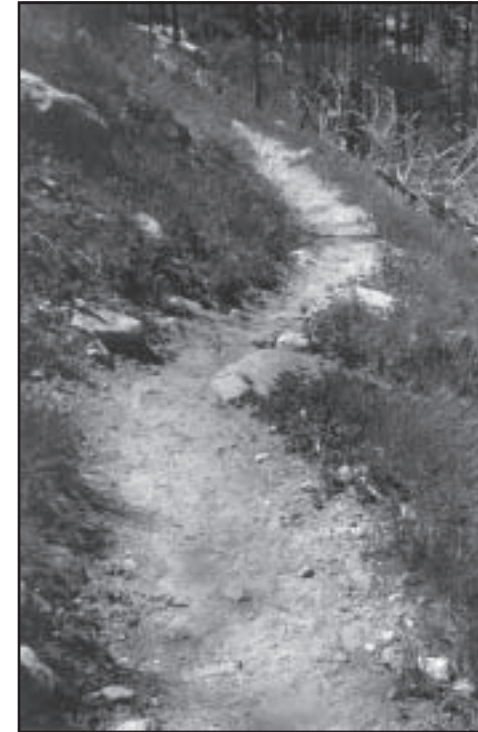
Figure 7—Rocks and logs help to keep the trail in place. And remember that this is a path through nature, not a monument to Attila the Hun.
