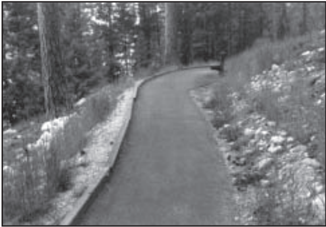
Figure 2—A smooth trail with a gentle grade is appropriate for an interpretive trail or a trail designed for easy access.
